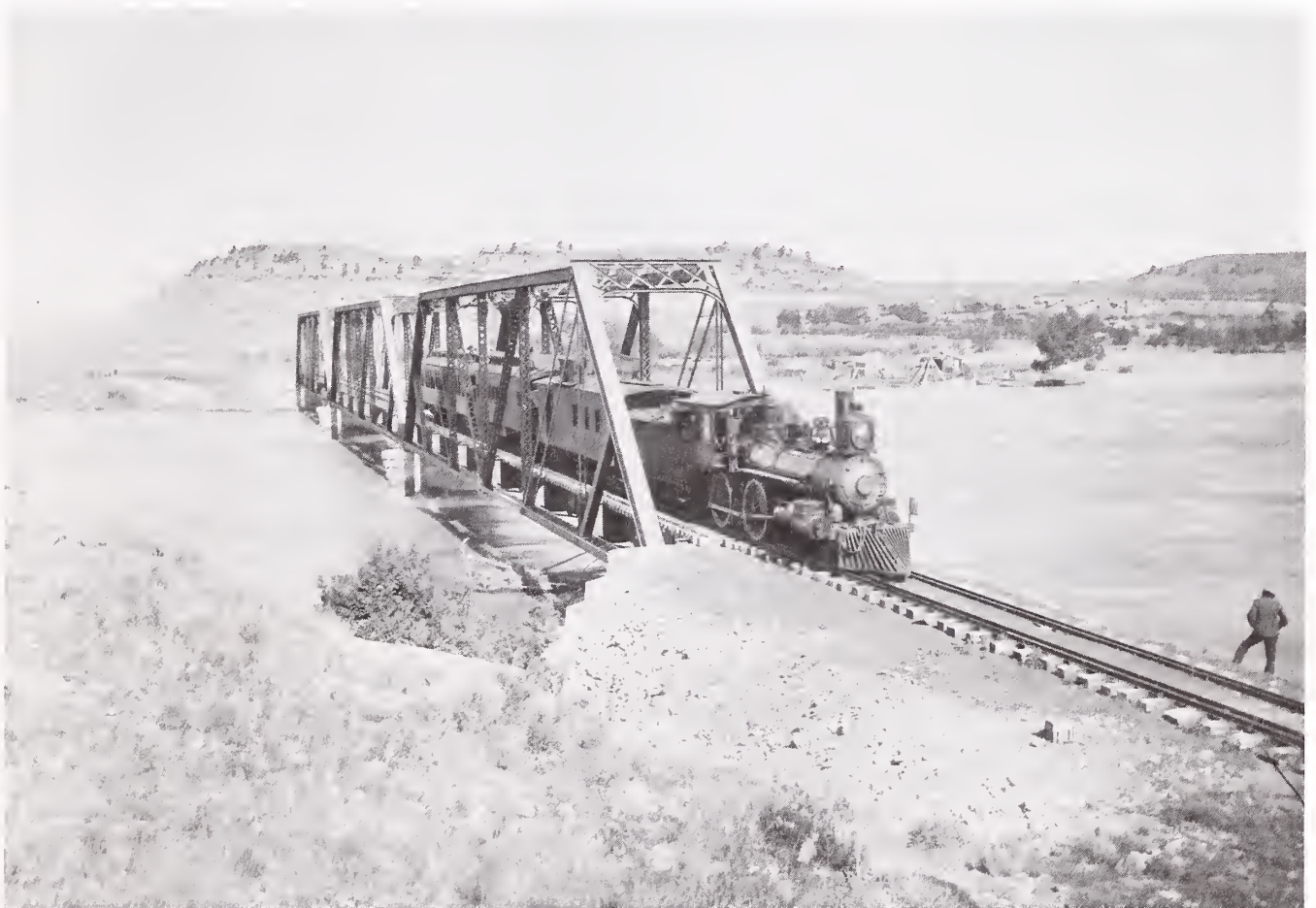
Northern Pacific Railroad Bridge over the Yellowstone River near Billings, 1894 (Haynes Foundation Collection. Montana Historical Society).
